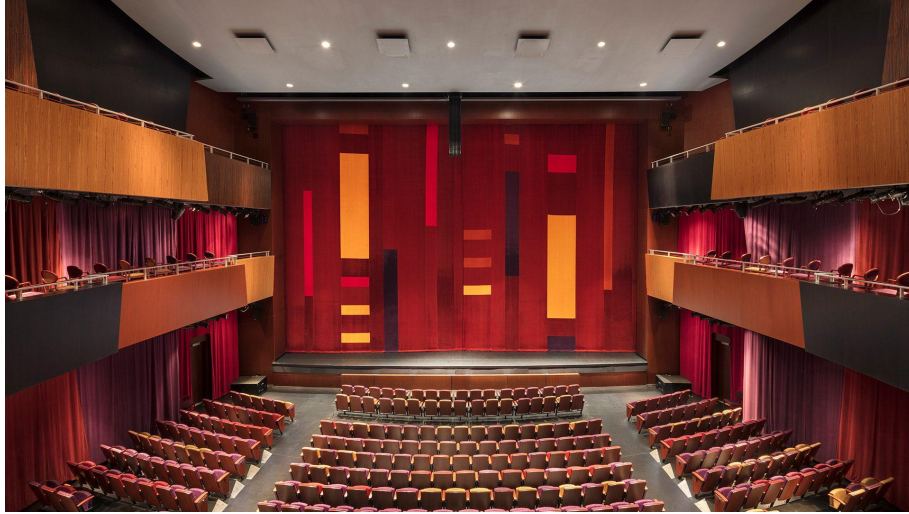
State-of-the-art, 961-seat performing arts space. The stage is a sprung floor built on rubber sleepers, 2- 3/4" layers of plywood topped with a black Masonite surface.
